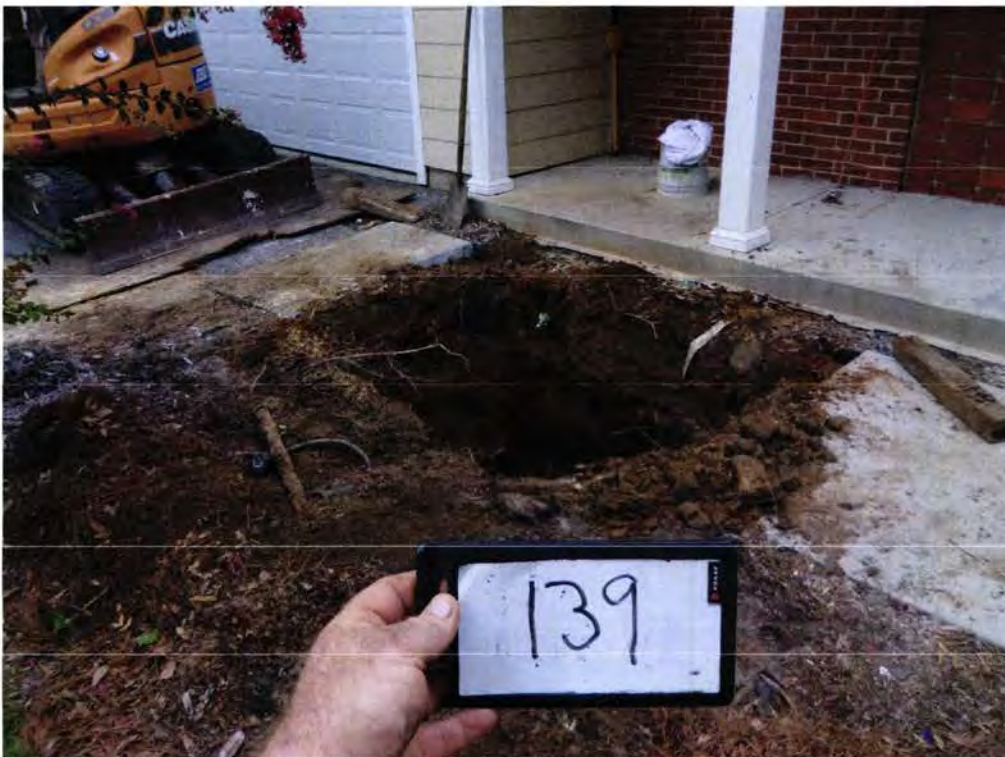
Picture 2: Excavation of UST 139LaurelBB.
